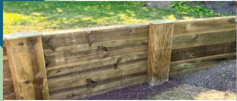
Retaining structure forming terrace also provides seating.
